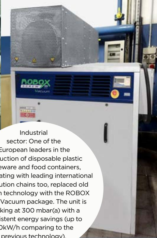
Industrial sector: One of the European leaders in the production of disposable plastic tableware and food containers, collaborating with leading international distribution chains too, replaced old vacuum technology with the ROBOX screw Vacuum package. The unit is working at 300 mbar(a) with a consistent energy savings (up to 30kW/h comparing to the previous technology).
