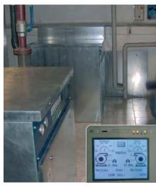
• Paper industry: Centralised vacuum systems ROBOX evolution pressurised blower unit in pressure (P) / air injection vacuum (DV)
