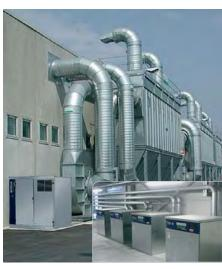
• Industrial: Pneumatic transport of wood chippings ROBOX evolution blower unit
